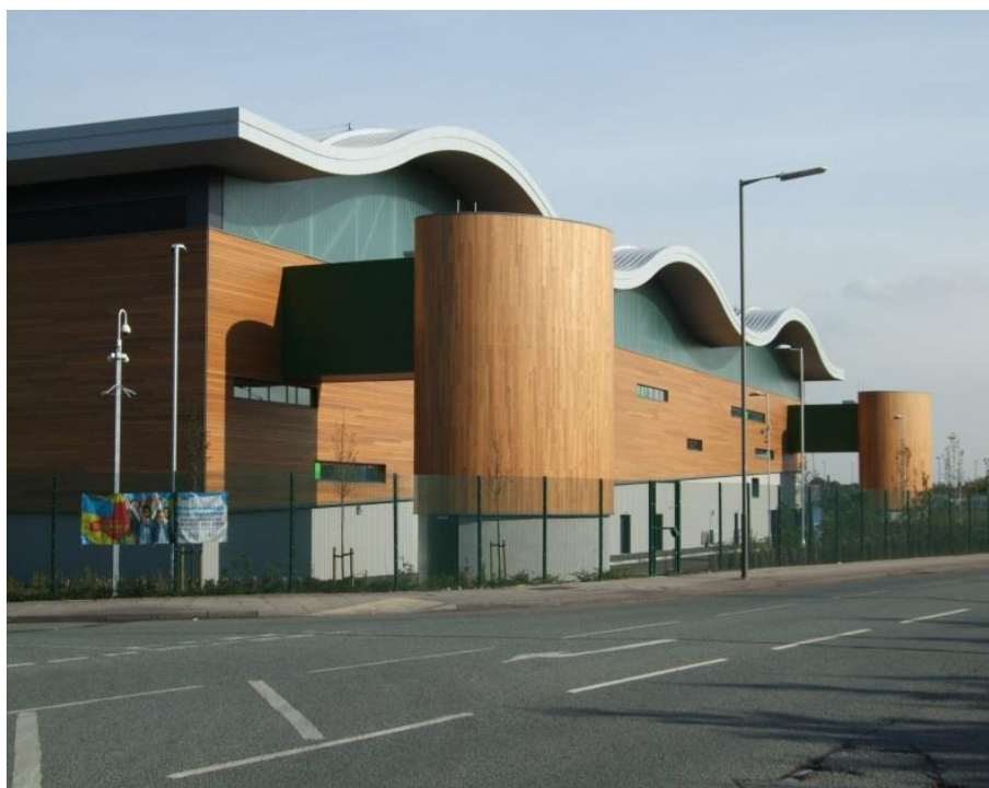
Photo credit: Merseyside Environmental Advisory Service
